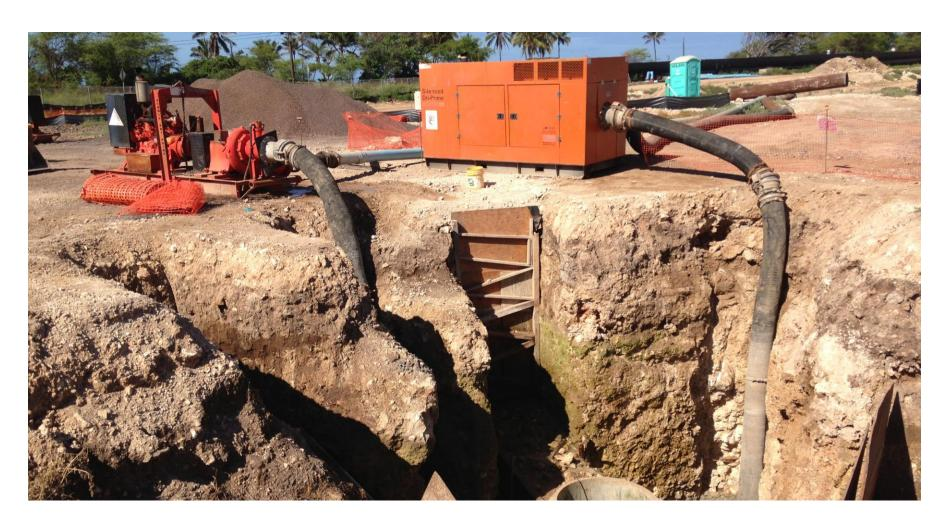
Delta Construction has been working to get all the ground work done for the Ka Makana at Hoakalei development in Ewa Beach. The past couple weeks Delta has moved about 20 million gallons of water from the excavation where they tied in the new sewer line and performed a 5.8 MGD sewer bypass to keep the line clear while they tied into it.
