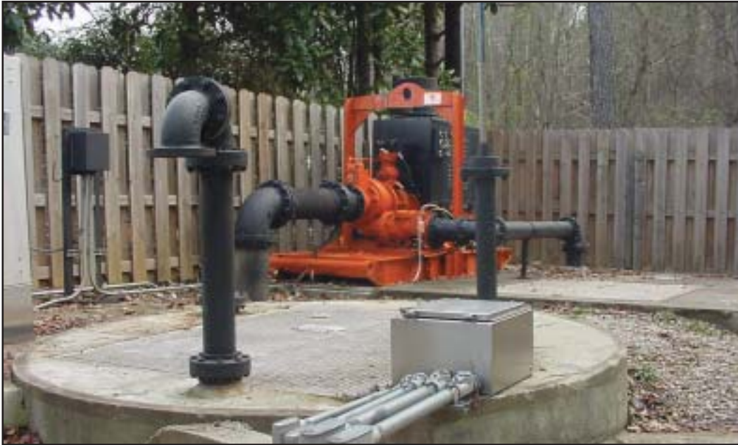
Godwin Dri-Prime pump with engine cover and locking door
