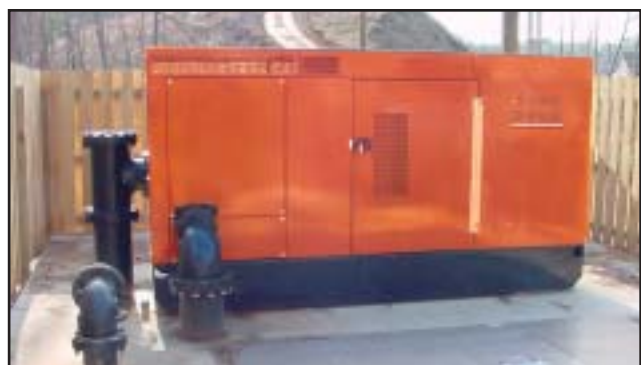
Godwin Critically Silenced Dri-Prime pump at City of Hoover, Alabama
