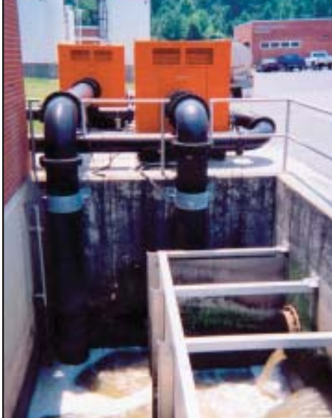
Two Godwin DPC300 Dri-Prime pumps at OWASA in North Carolina
