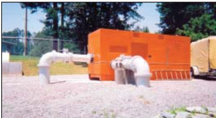
Godwin HL10M Dri-Prime pump at OWASA in North Carolina
