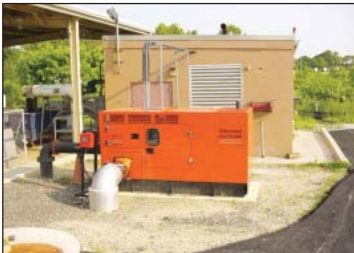
Godwin Critically Silenced Dri-Prime pump in Jessup, Maryland
