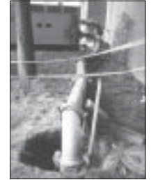
CD150M 6" (150mm) Dri-Prime for Stormwater Sewer Bypass
