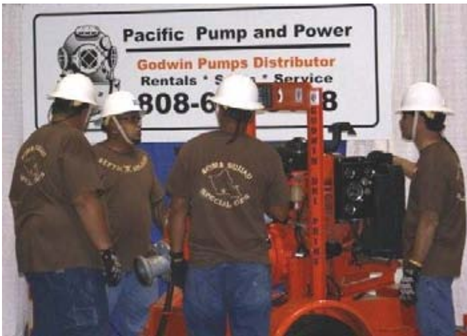
Maintenance Challenge: The teams prepare a Godwin Dri-Prime CD100M for service at a disabled lift Station.
